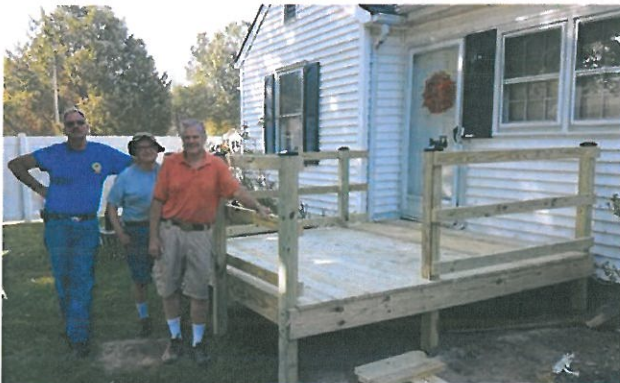
Another Handicap Ramp Completed at 49 Rens Road.
